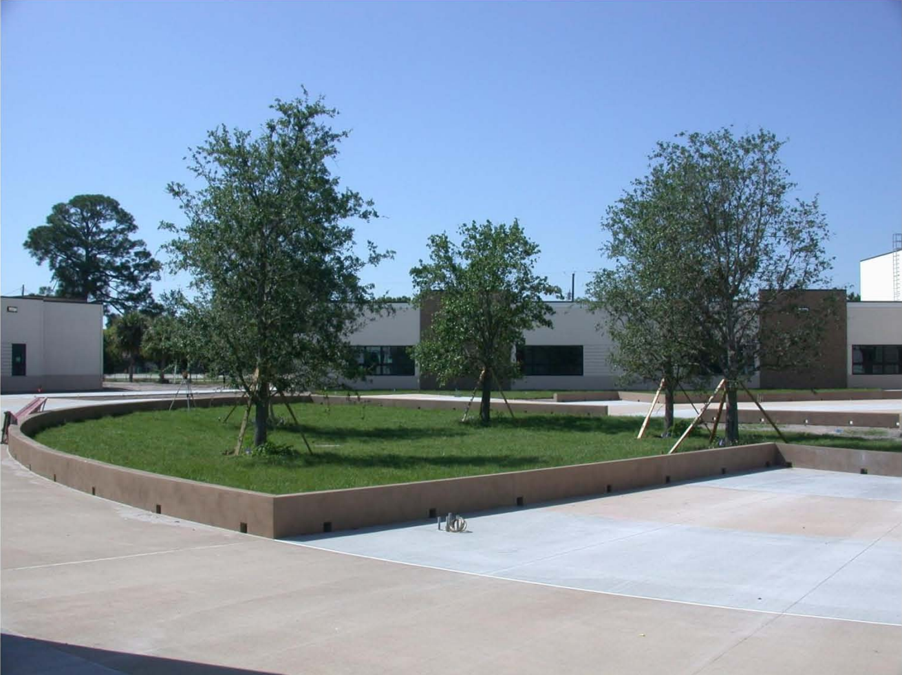
Vero Beach Elementary: Courtyard View to the South
